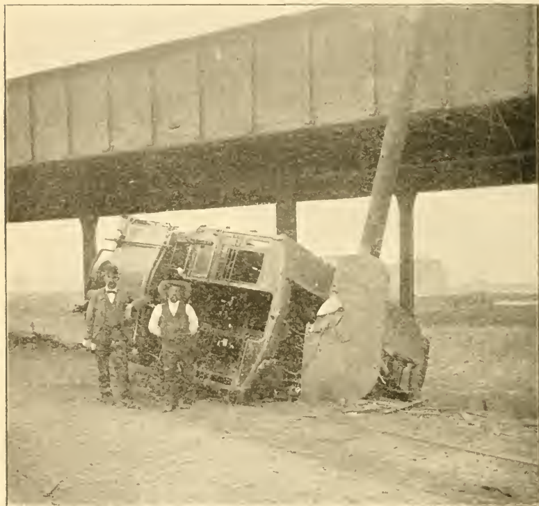
EAST ST. LOUIS ELECTRIC CAR BLOWN FROM THE BRIDGE.
